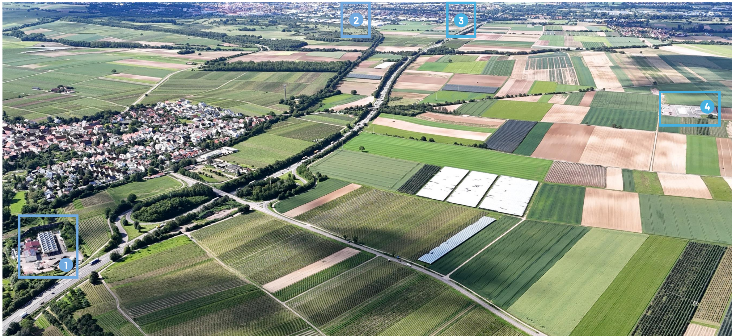
1 Vulcan's 100% owned Insheim Geothermal Power Plant (operating)
